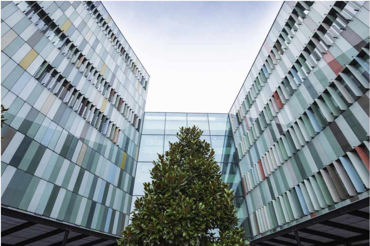
Eurotecnica office, Milan, Italy
