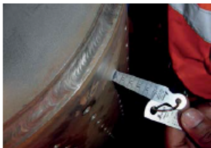
Inspection of equipment internals.
