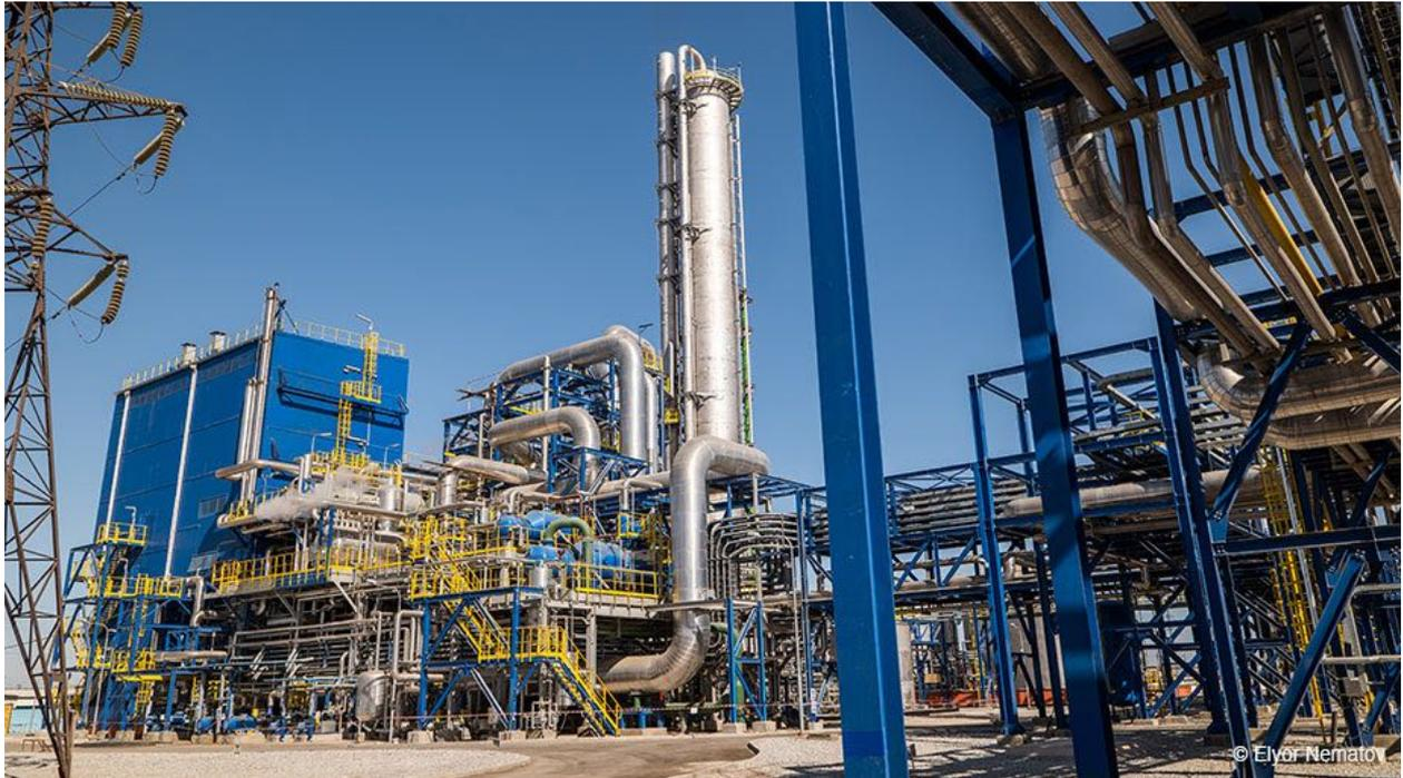
*Nitrous gas reacts with water inside the 50-meter absorption tower, producing nitric acid. Casale's use of an extended absorption column design reduces ammonia slippage and emissions.*
