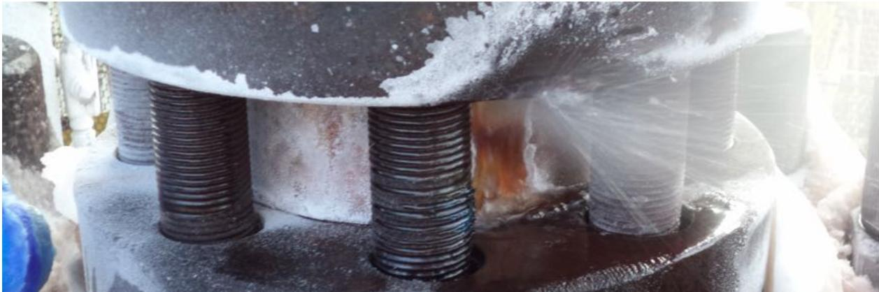
**Figure: A leaking flange connection**
