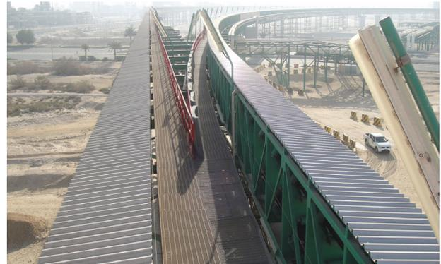
Figure 7 – Interconnecting Pipe Rack (ICPR) between the QAFCO Sites
