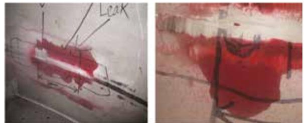
Figs. 9 & 10: (Leakage Area) & (Pinpoint Location)
