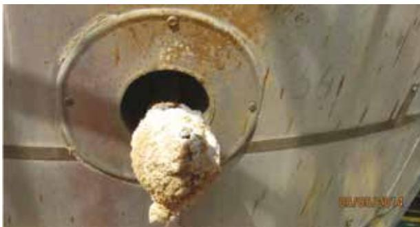
Fig. 3: (Leakage through Weep hole)
