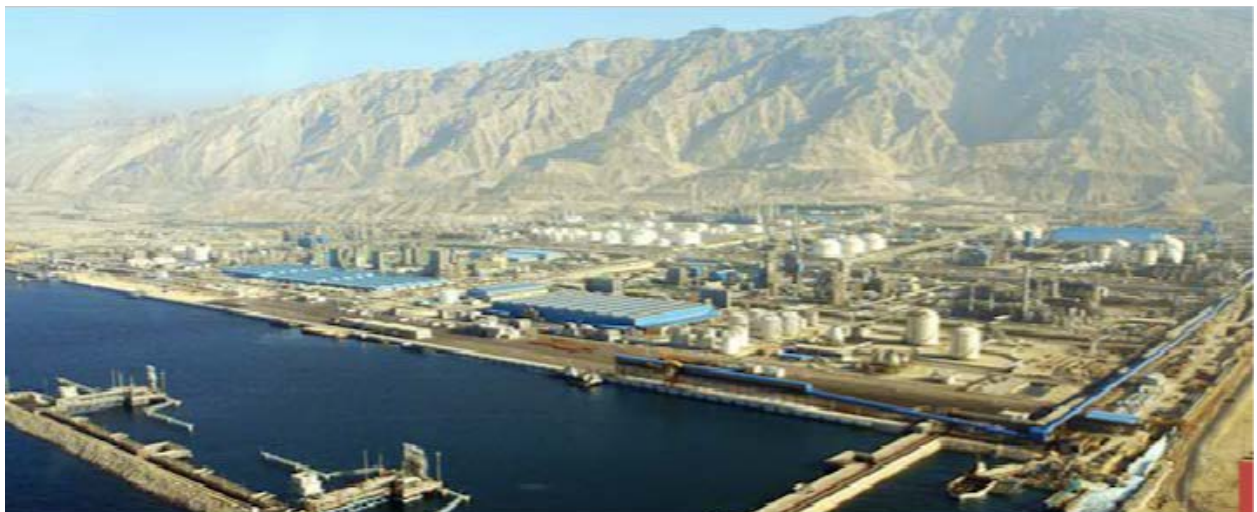
Figure 2: Site of Pardis Petrochemical Company
