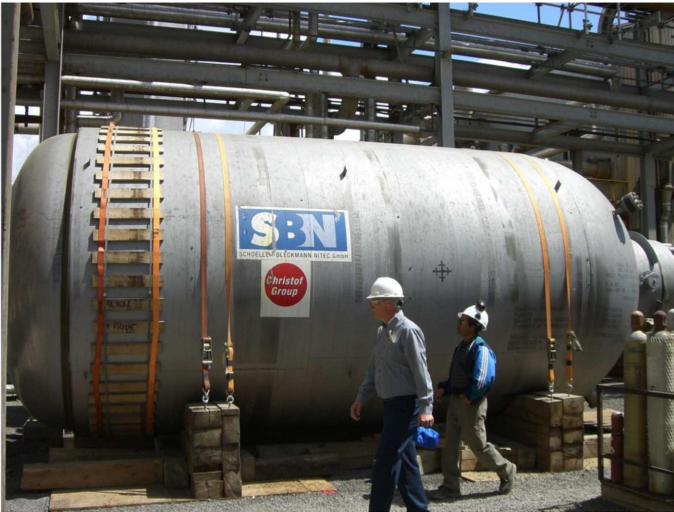
*Figure 2: New top reactor shell section*
