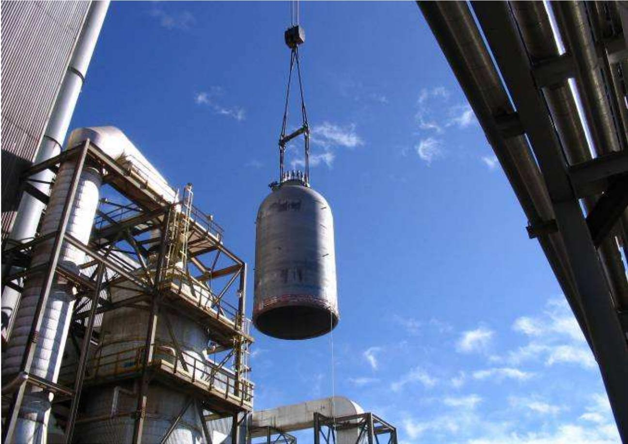
*Figure 5: New reactor section being lifted*
