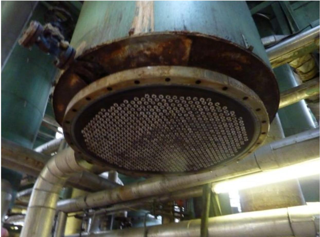
Another advantage of installing a restriction orifice in each tube over an orifice plate is that there is no risk of bypassing and mal distribution. Finally, the costs of these restriction orifices are significant lower.
