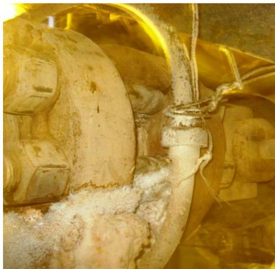
Fig (iv): Air Sparge over Leak Flange
