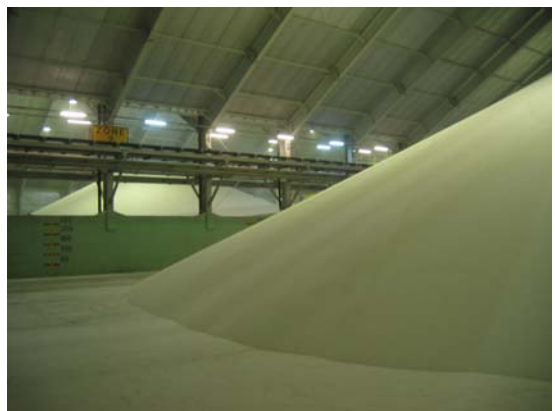
Figure 2 - Urea storage warehouse showing angle of repose
