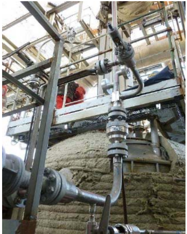
Figure 9, 10, 11: Installation and welding in of Pre-fabricated spools
