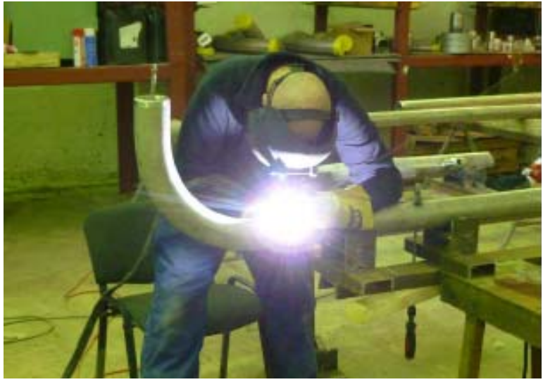
Figure 8: Welding of a 6 inch bend
