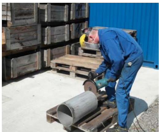
Figure 5: Cutting of pipe
