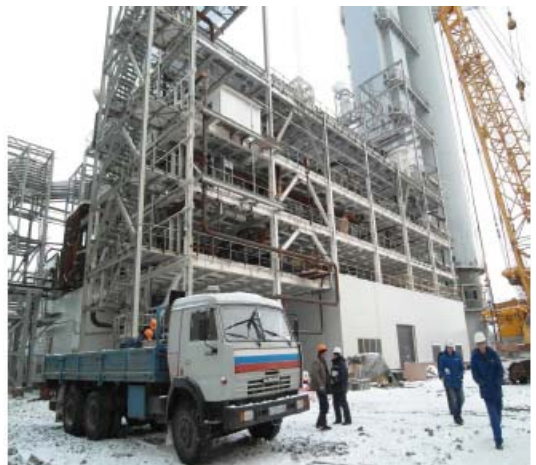
Figure 3: Finished steel structure
