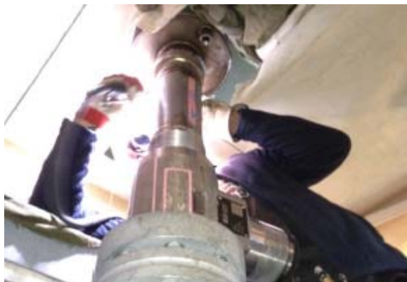
Figure 9, 10, 11: Installation and welding in of Pre-fabricated spools
