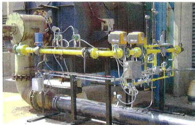
▲ **Figure 2.** Before pressure testing, make sure that all equipment is properly isolated. Verify that all main equipment shut-off valves are closed and are able to hold pressure. Otherwise, regulators and other sensitive fuel train components could blow out.
