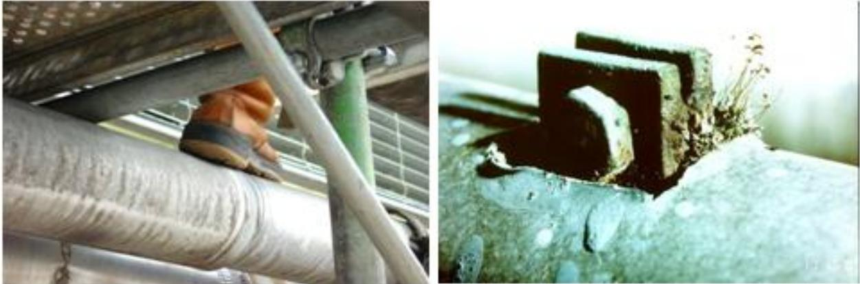
Further with austenitic stainless steels one has to pay proper attention to chlorides as these can cause chloride stress corrosion cracking. Using glue or paint containing chlorides can cause already trans-crystalline cracks as in the flange face indicated in the picture below.
