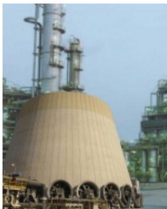
Part of the Safco 4 plant is a cooling tower to cool down the sea water taken from the Arab Gulf. This shows the strict environmental regulations which are valid in this region. The ammonia plant is a Uhde license and has a design capacity of 3300 mtpd. Its start up experiences has been presented at the 20<sup>th</sup> AFA International Annual Technical Conference Tunisia 2007.<sup>11)</sup>
