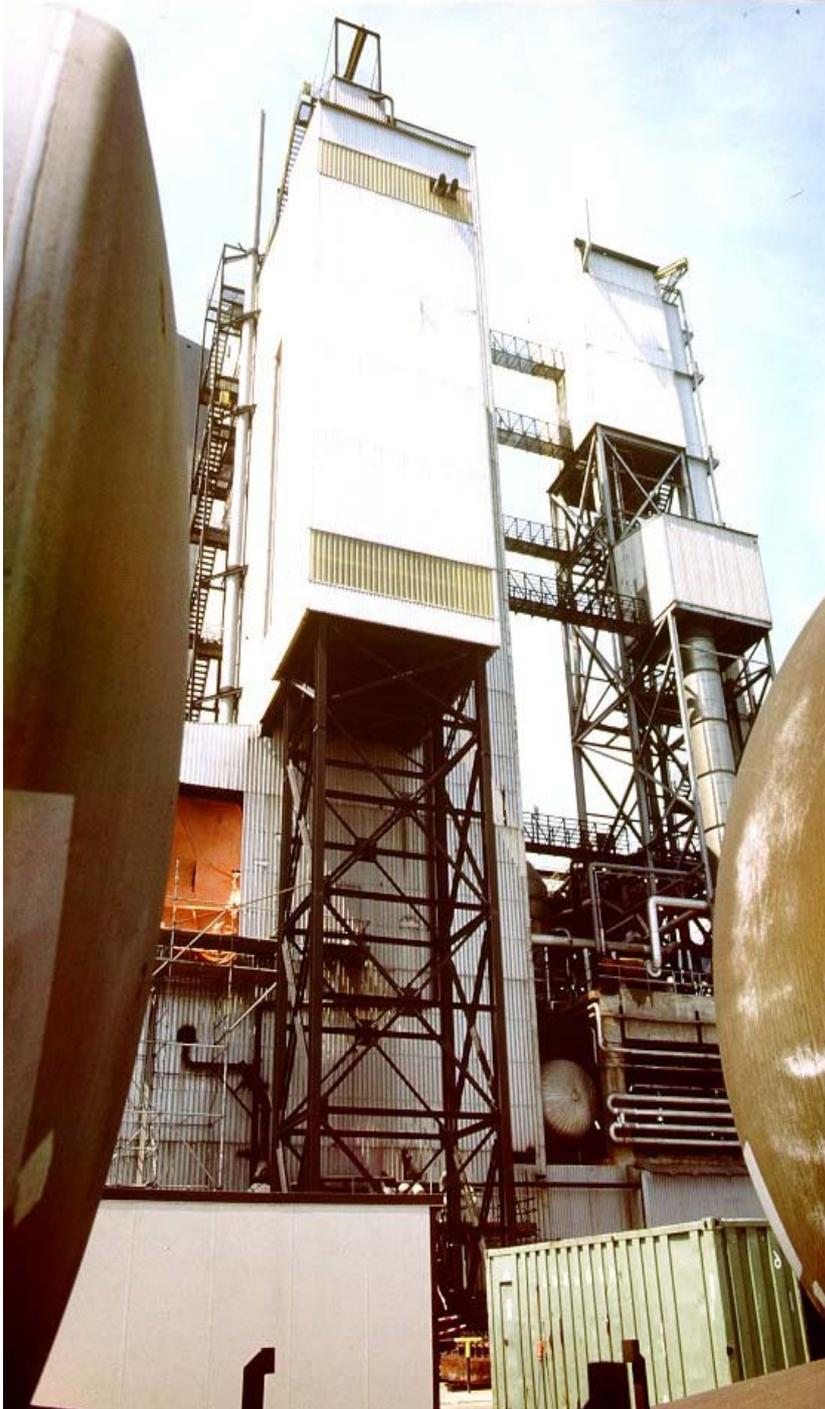
**Photo 2: Indoor design of HP equipment of urea stripper plant by means of aluminium cabins**
