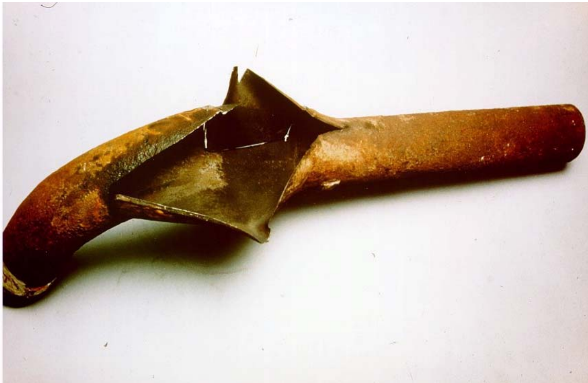
Photo 1: Atmospheric corrosion in HP CO 2 pipeline from urea plant.
