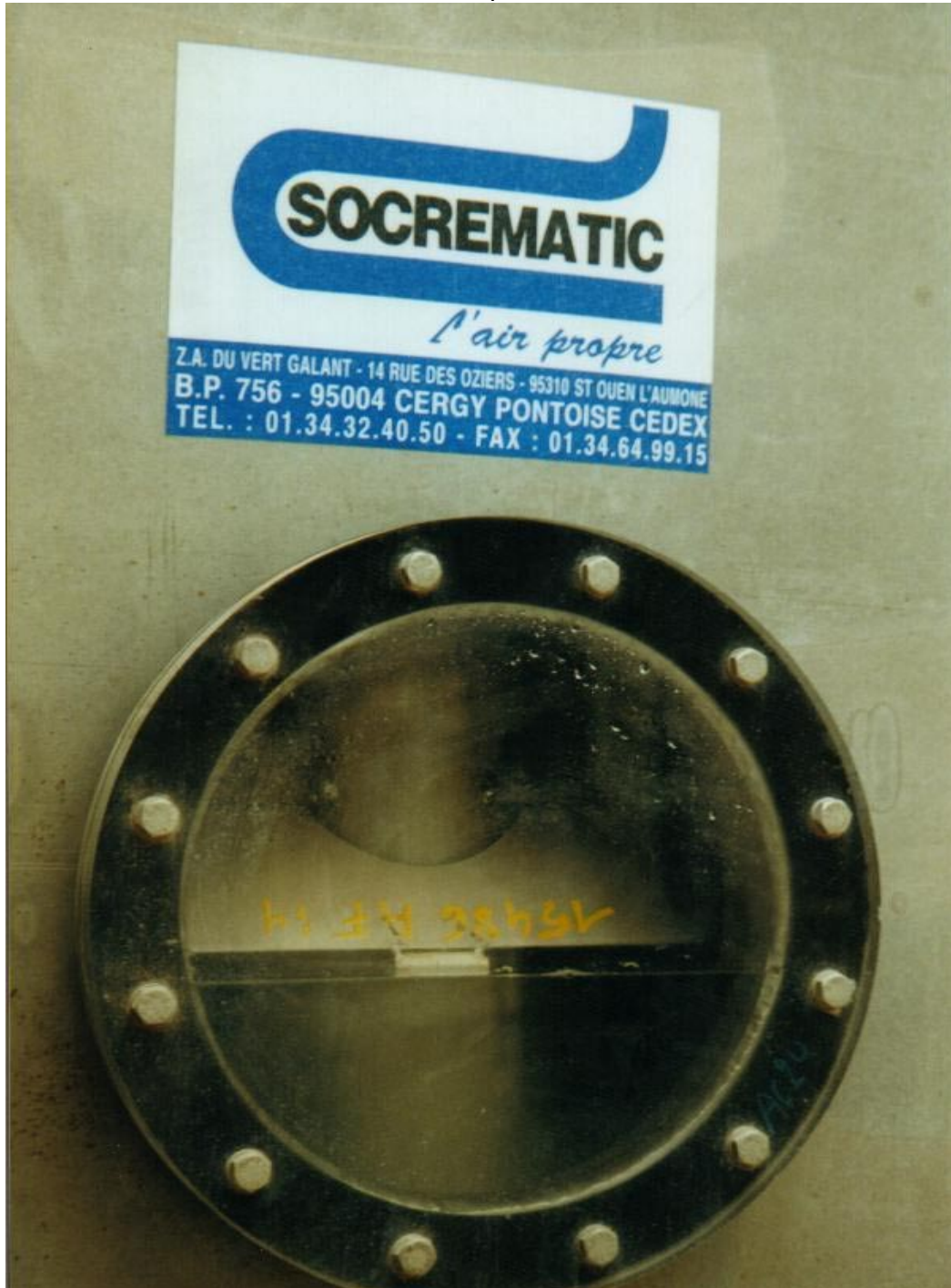
ADJUSTABLE SLIDE PLATES ON THE ANNULAR SKIRT PRIOR TO OPERATING (OUTSIDE VIEW)
